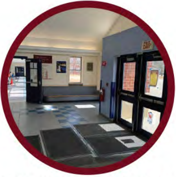
SAFETY & SECURITY CONCERNS
